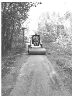
Sweco mini-dozer and Skidsteer were used for cutting the new trail corridor and moving the sod from the new trail to the old trail for its rehabilitation. DNR Parks and Trails crew have amazing skills with these machines.
